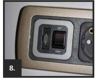
8. SWITCH OFF HEATER ISOLATION SWITCH
