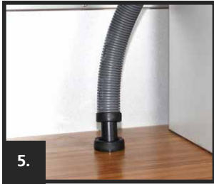
5. WASTE PIPE FITTING
