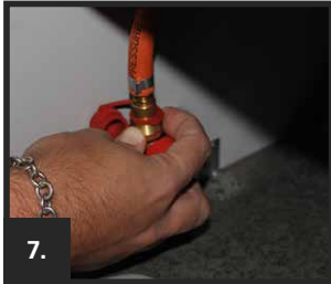
7. ONCE GAS IS TURNED OFF PUSH DOWN ON BRASS NECK
