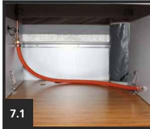
7.1 PULL THE HOSE FROM UNDER THE KITCHEN BASE UNIT
