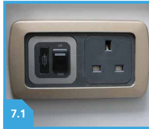
7.1 HEATER ISOLATION SWITCH
